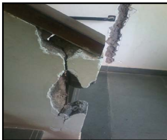
Pic: Walls of the college walls after drilling
